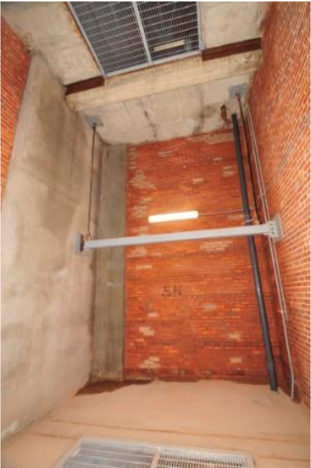
Level E is one floor below the bell chamber. New structural steel reinforcement was added along with new lighting, electrical conduit, galvanized grating and the storm drain.
