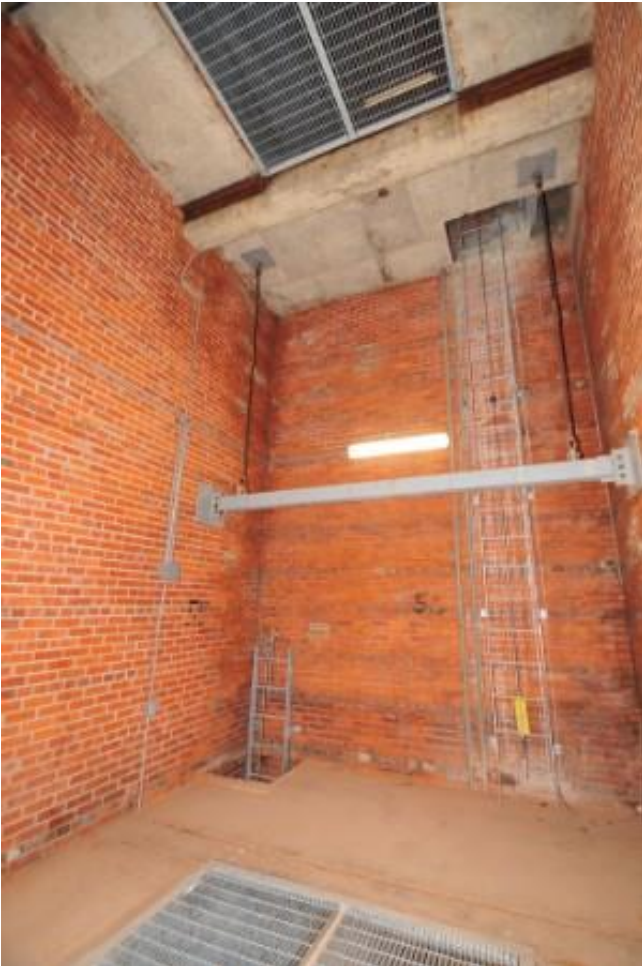
Level E is one floor below the bell chamber. New structural steel reinforcement was added along with new lighting, electrical conduit, galvanized grating and the storm drain.
